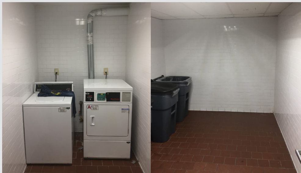
The City’s Shelter Repair Squad retiled the laundry and refuse rooms at the Win Liberty Family Residence.
